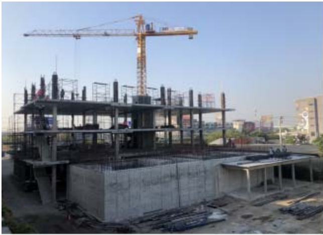
Ex 10: Construction Progress Of Cancer Center
