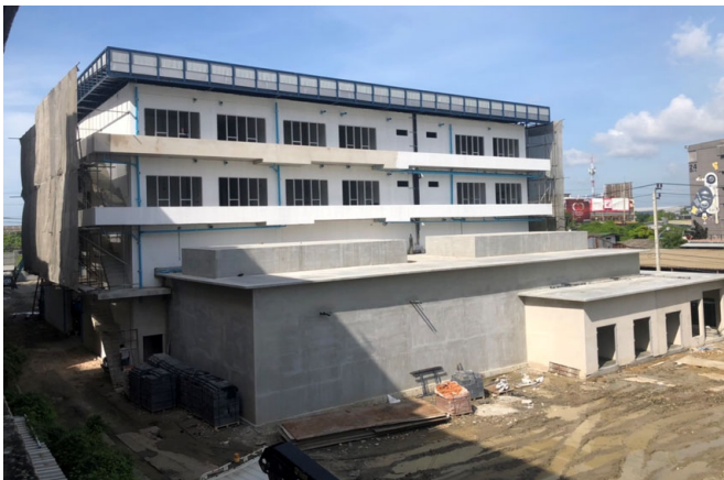
Ex 7: Shewarat Cancer Center – Construction Progress
