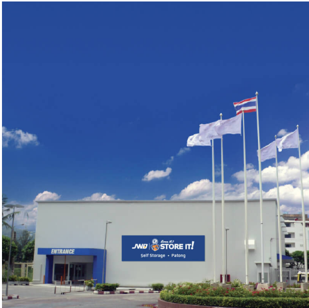
Ex 4: Store It! Patong (Phuket) Branch
