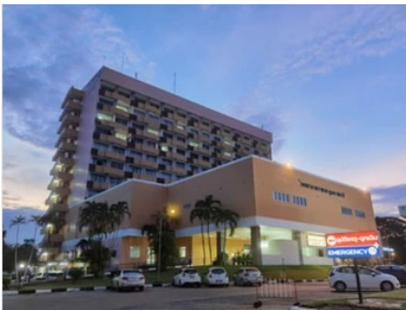
Ex 8: Rajavej Ubonratchathani Hospital
